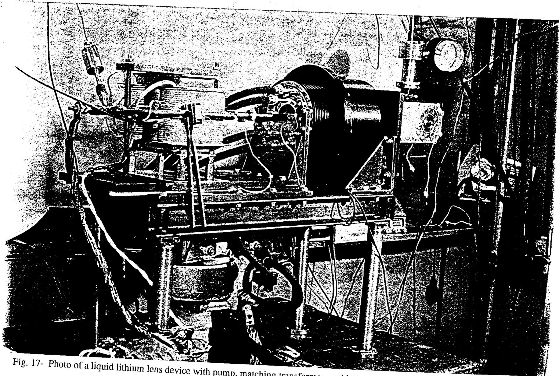
Fig. 17- Photo of a liquid lithium lens device with pump, matching transformer, and heaters.
