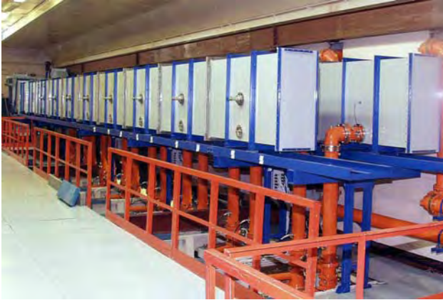
Fig.6: RF power division system
