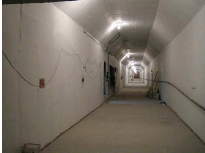
Figure 11: A 800 m tunnel for 2.5 GeV linac.
