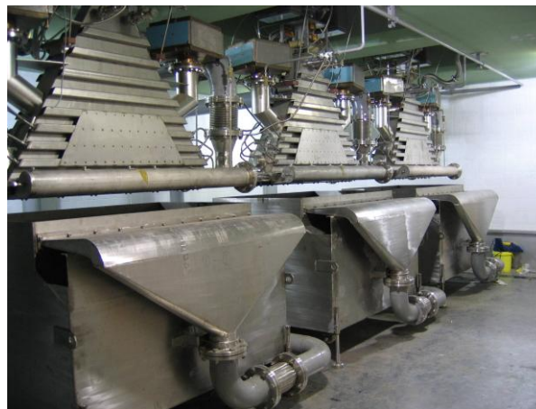
Figure 7: Irradiation hall for wastewater treatment with ELV-12 accelerator.
