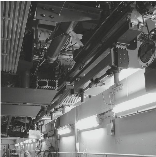
Fig. 6. The third stage FEL undulator sections.
