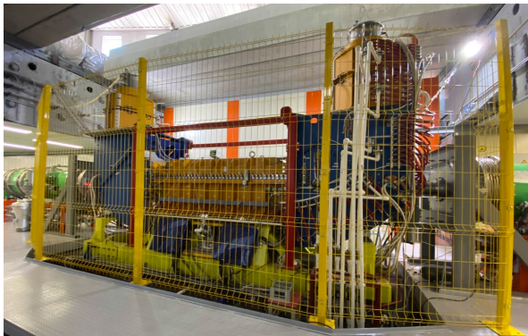
Figure 2: Booster electron cooling system.
