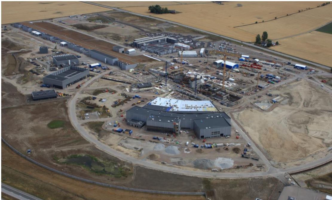
Fig.1 The Photo shows a recent view of the ESS construction site.
