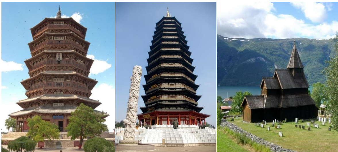
Fig. 2. Tianning Pagoda of temple complex; Sakyamuni Pagoda of Fogong temple; Urnes stavkirke in Norway
