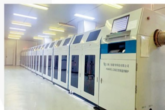
↑MOD facilities for superconductor layer
