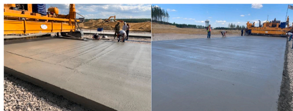
Fig. 1. Cement concrete road construction.
